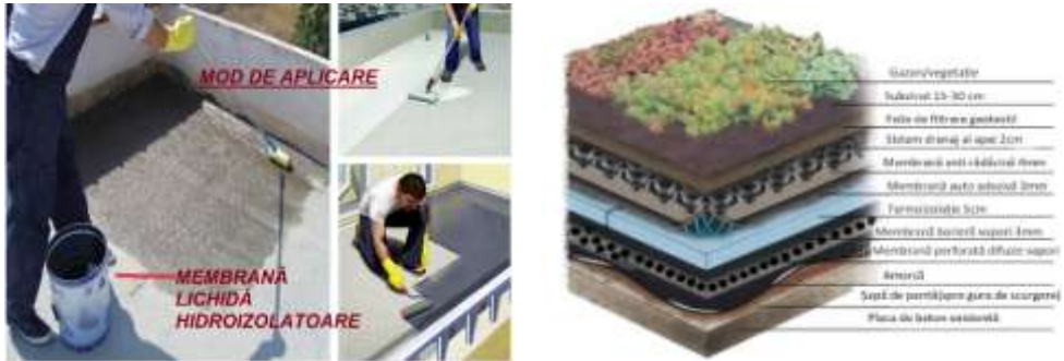
Fig. 3. Isolation layers of the terrace
